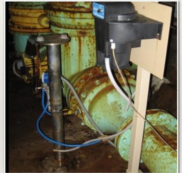
Existing Filter Piping Conditions
