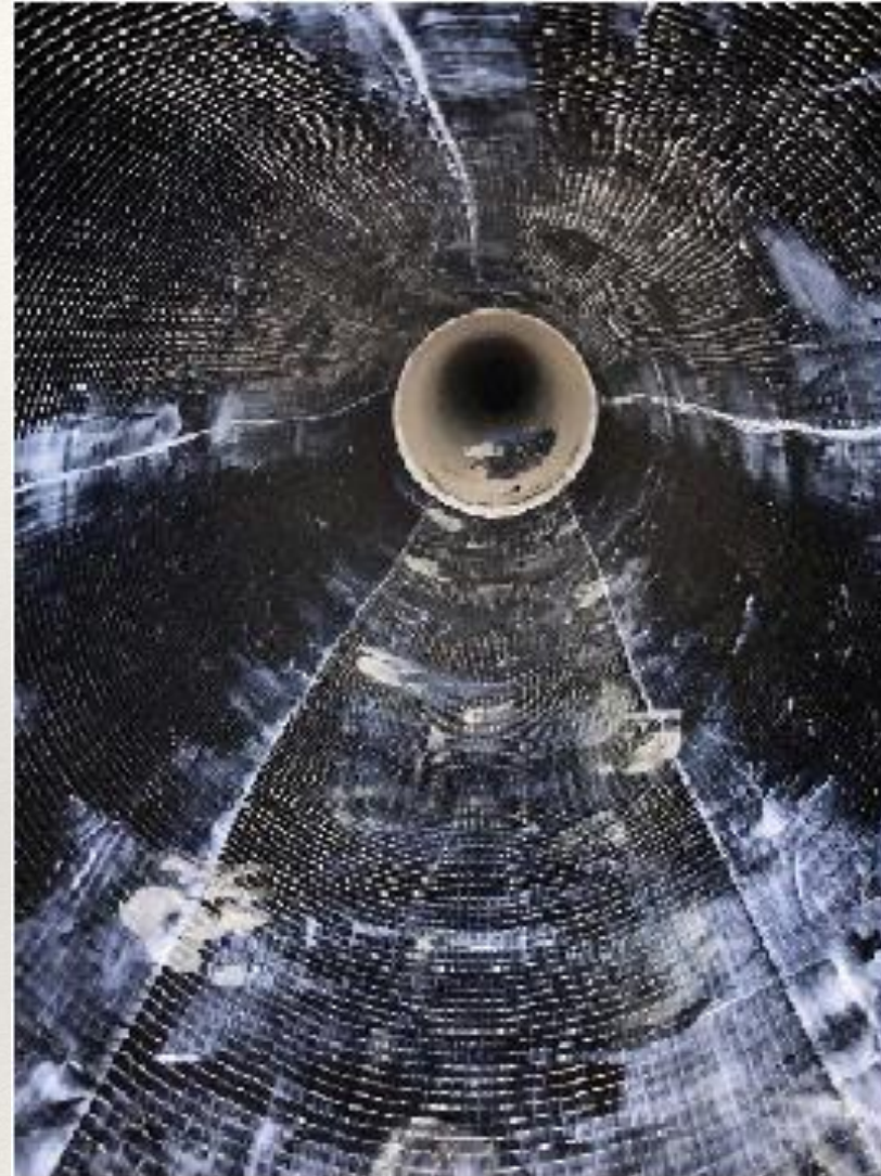
Figure 1 – Second Cured Layer of CFRP.
