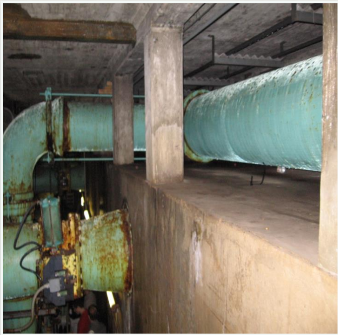
Hydraulic Valve Actuator Corroded Leakage
